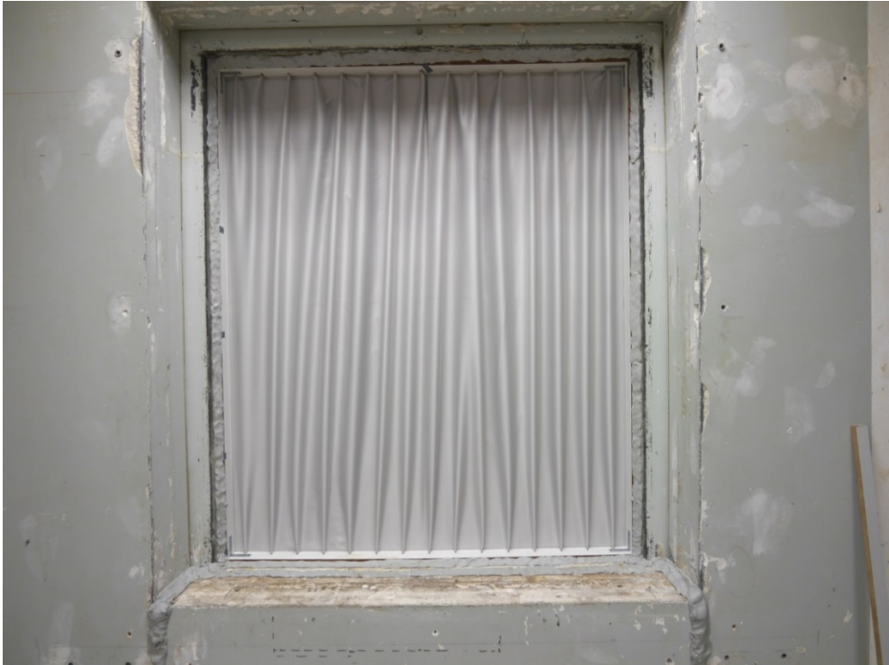
Figure B.2. Exemplary picture of a specimen in the window test stand (source room side).
