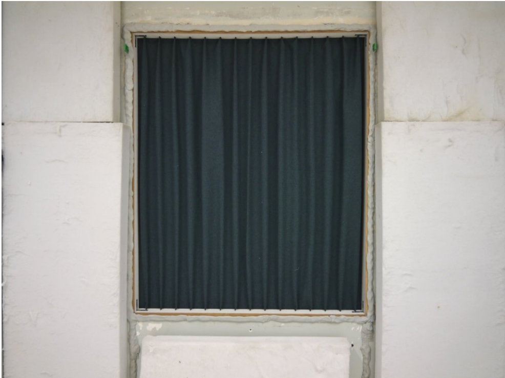
Figure B.1. Exemplary picture of a specimen in the window test stand (reception room side).
